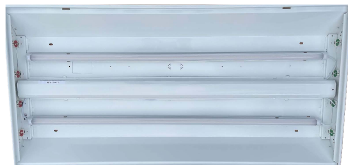
2x4 LMK retrofit completed with ballast cover replaced.
